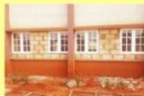
UNSS classroom renovation
